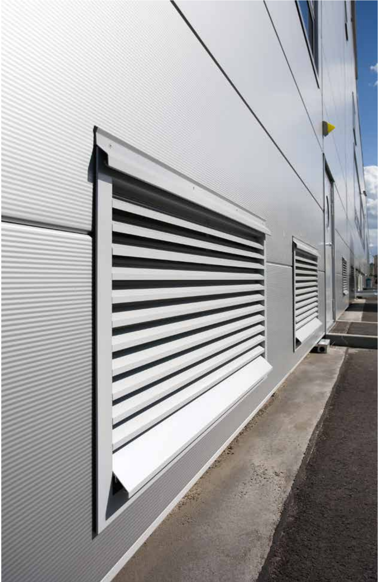
Built-in wall louvre, heavy-duty series 481 (see p. 50)
