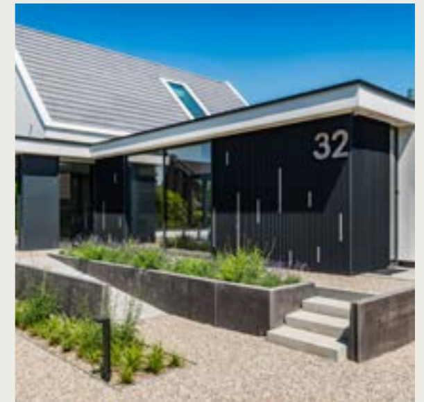
Inserts with wood and LED modules
